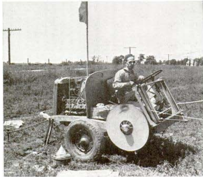
This is another view of the power winch with operator at his post
